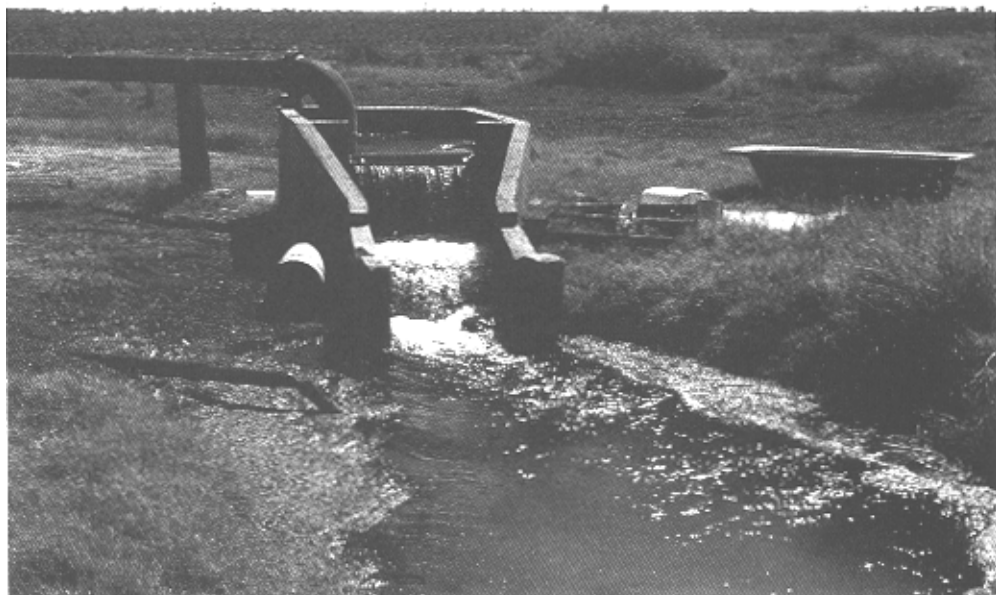
Artesian bore and drain
