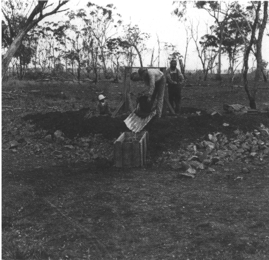
Hand digging a well at the turn of the century.
