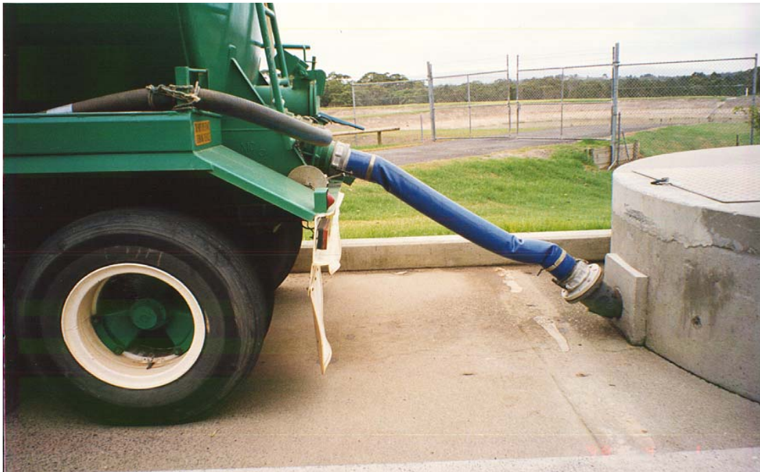
Figure 7: Tanker unloading effluent through flexible connection and KAM-LOK coupling
