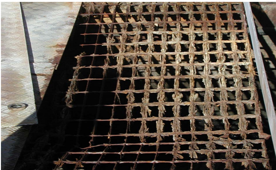
Effect of high strength and low pH waste on sewage treatment works
