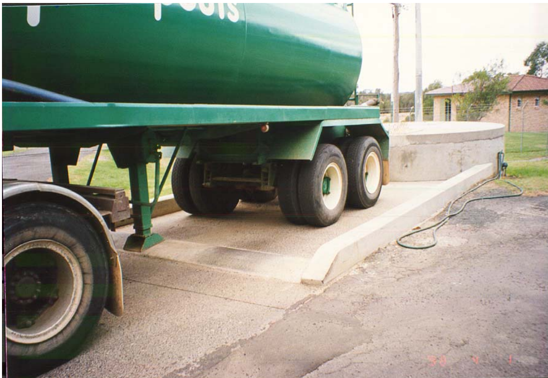
Figure 8: Loaded tanker in bunded area which drains into holding tank
