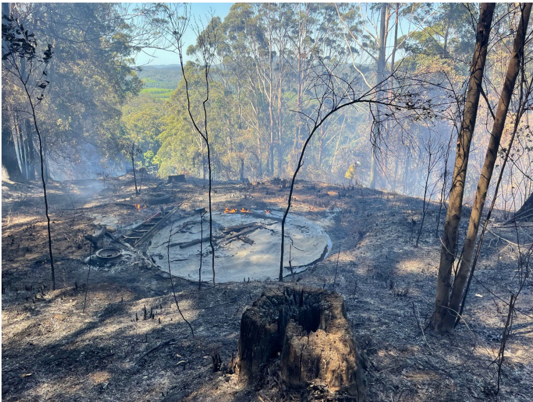
Image: Burnt water tank on a NSW north coast property. Photo credit: Vivienne Nehme.
