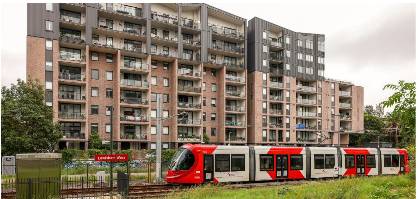
Mid-rise housing and inner city transport, Summer Hill, Sydney. Image credit - James Grabowski/DPHI
