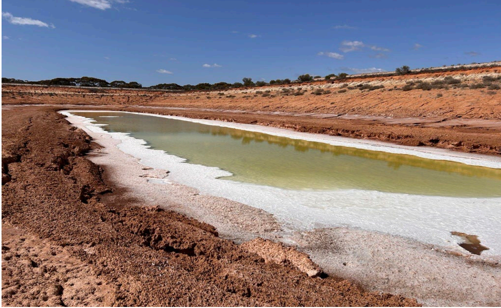
Figure 4-2: Erosion and siltation of the Mallee Cliffs SIS enhanced leakage pit (photo D Lalor 2024)
