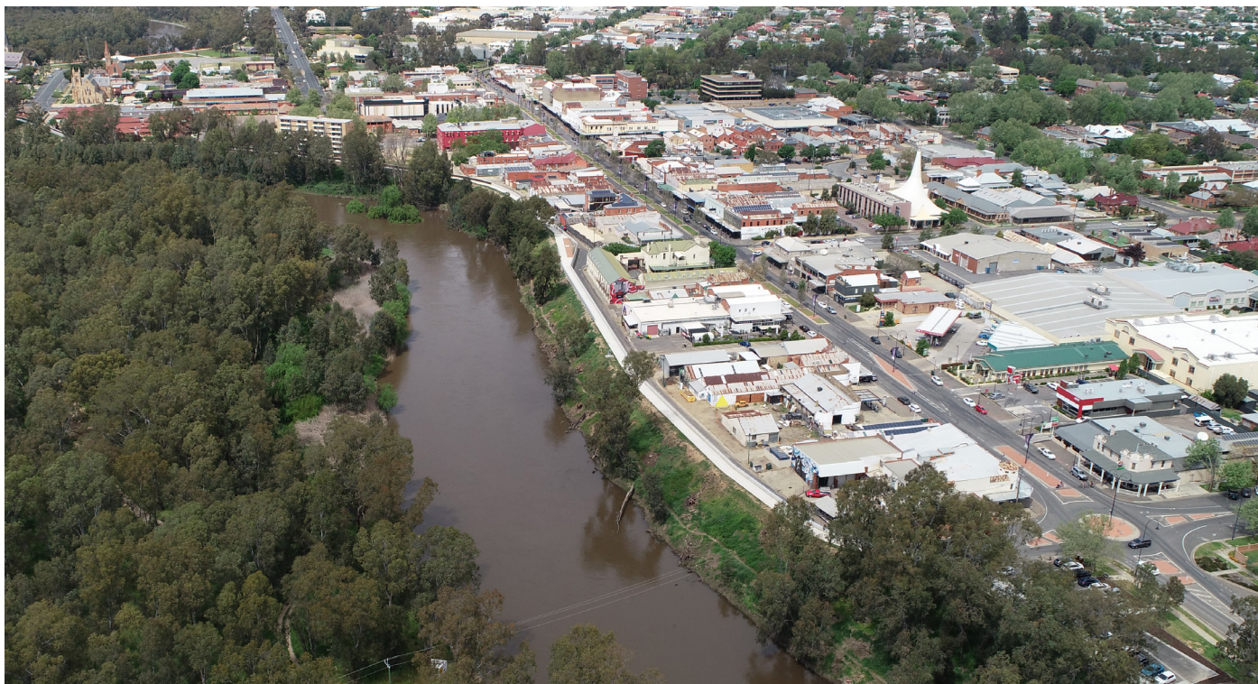
Wagga Wagga Murrumbidgee River levee bank
