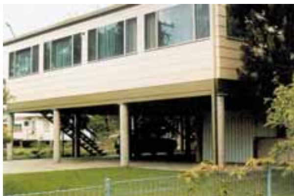
PLATE 9 - Flood Proofed by Raised Floor Level
