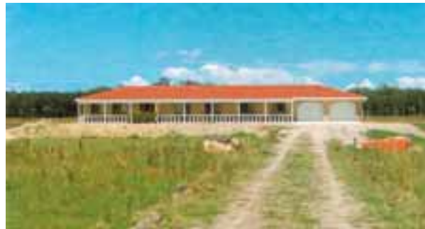
PLATE 12 - Flood Proofing with Fill
