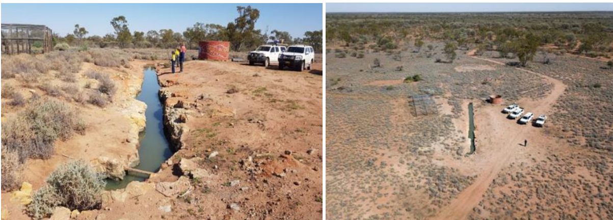
Figure 46: a) Old Gerara Spring showing long excavated pond and metal bar across channel, and b) aerial view of spring site (DPIE, 2020b)
